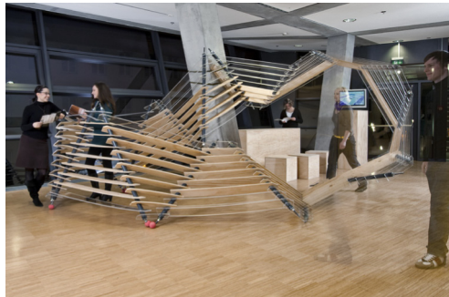
Figure 9 Moebius strip with ribs within planar trapezoids
